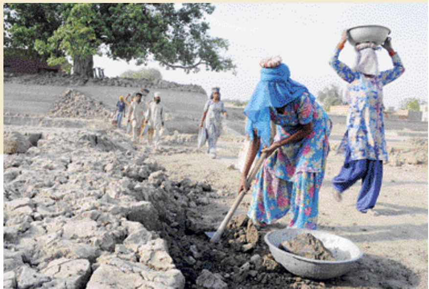
Labourers digging a pond
